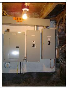
These two panels are the main breakers that will cut power from the building. They are located in the basement, over from the far right wall (Main Street side of building)
