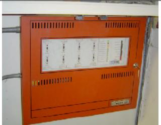
Fire Alarm Panel. Eight zones identified. Periodically check to make sure Fire Alarm Panel is functioning properly
